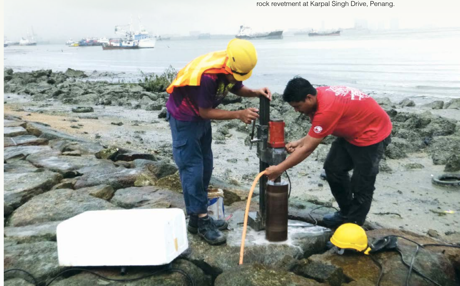
The drilling of artificial rock pools on the newly constructed rock revetment at Karpal Singh Drive, Penang.
