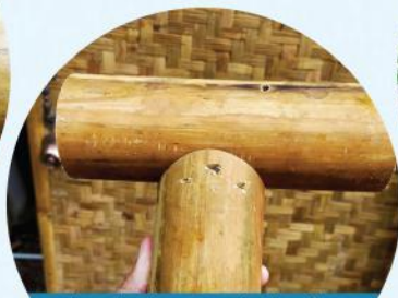
Pilot holes made before jointing bamboo with nails
