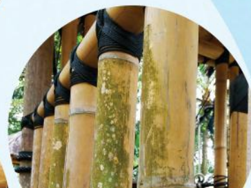
Mould, fungi, and algae on bamboo structure
