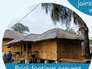
Brick footings prevent bamboo from direct contact with soil
