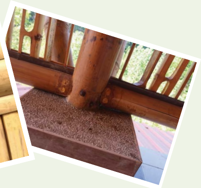
Bamboo jointing strengthened by using rope and nails
