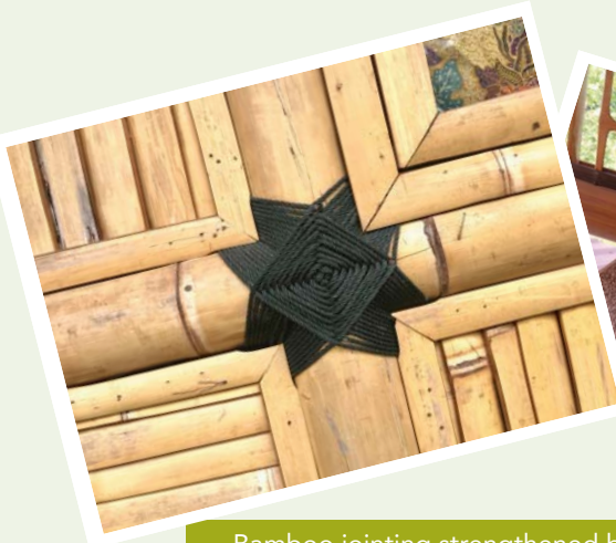
Bamboo jointing strengthened by using rope and nails
