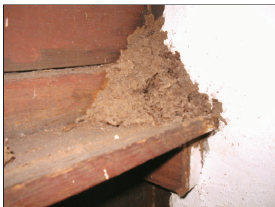
Fig. 28. M. crassus infestation on external structure of a house.
