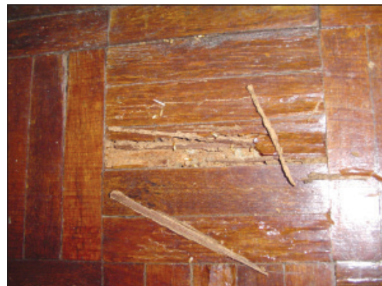
Fig. 7. Parquet floor infested with C. gestroi .
