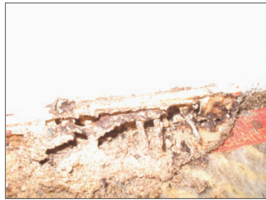
Fig. 5. Carpet grippers infested with C. gestroi .
