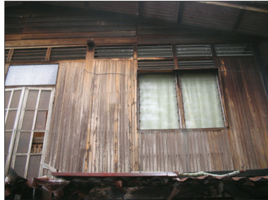
Fig. 23. Nasutitermes sp. infestation on external wooden wall.
