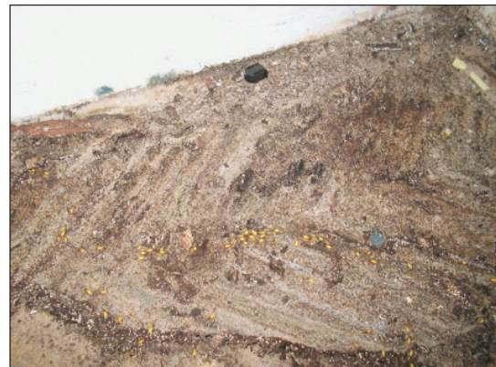
Fig. 19. G. sulphureus infestation under the carpet.
