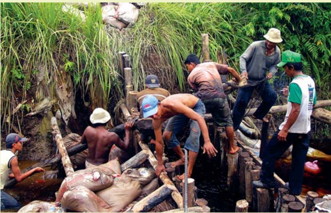
Community folks working together to block the canal for fire prevention in Riau, Indonesia
